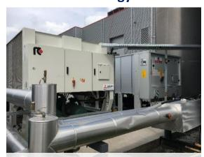
Mosonmagyaróvár 2 RC EVO FREE chiller Cooling capacity: 1200 kW
