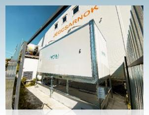
Pesterzsébet MITA MCC closed circuit cooling tower 950kW capacity
