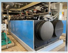
Budapest TX-W 1A00-6D00 water cooled chiller 2 x 3,5 MW
